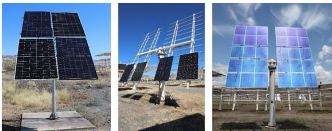
Figure 23 Testing facilities installed on the PSA for the comparison of the different PV technologies.
