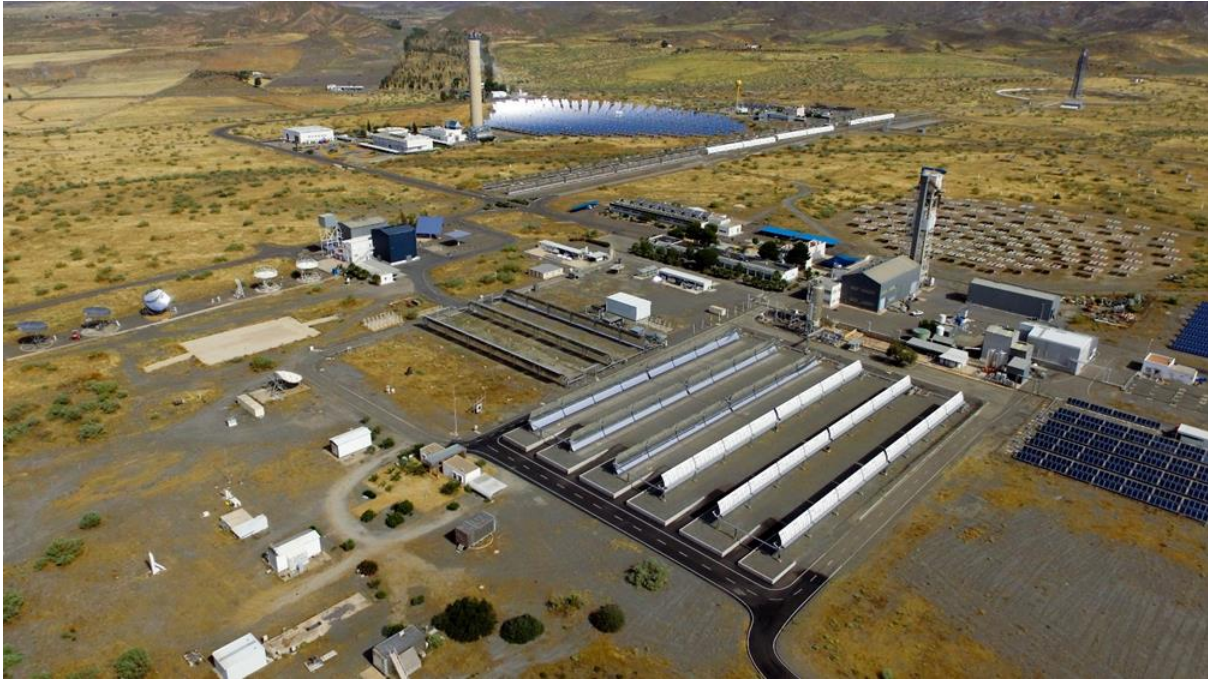
Figure 2. Aerial view of the PSA
