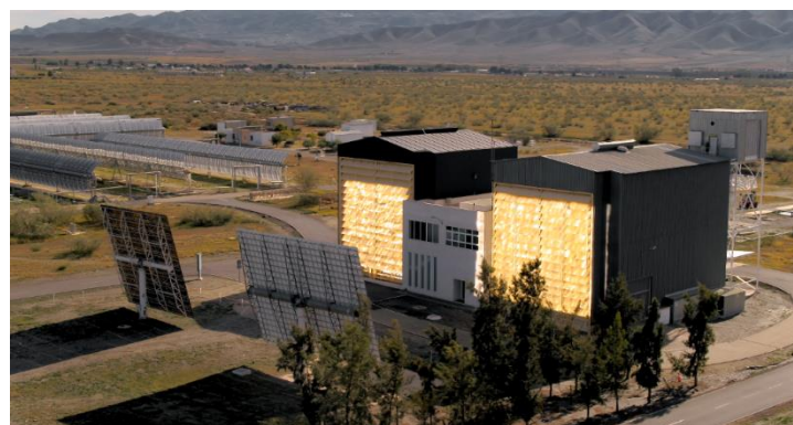
Figure 33. The three PSA solar furnaces. The SF-60 is the one on the bottom right.
