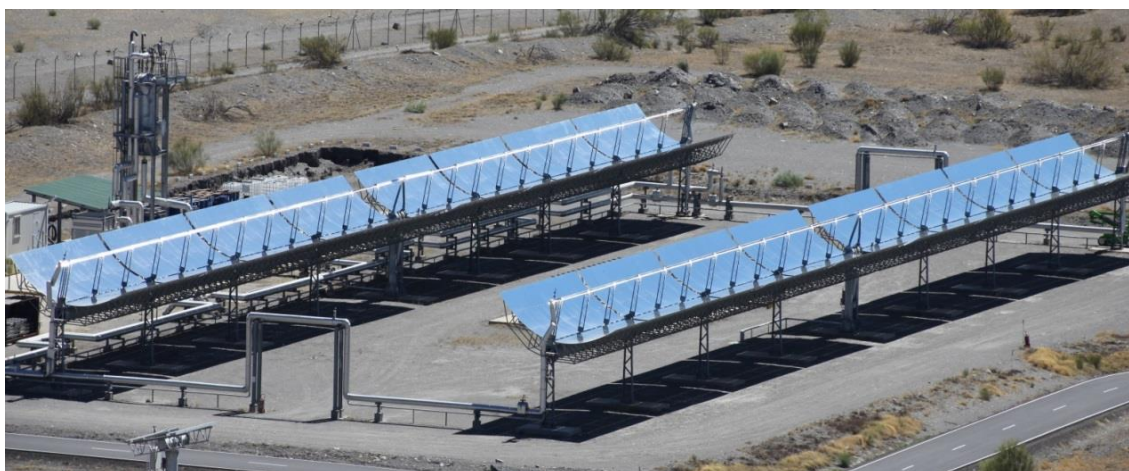
Figure 55. View of the PROMETEO test facility.
