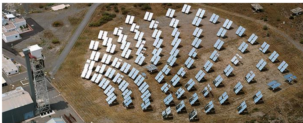
Figure 66. Aerial view of the experimental SSPS-CRS facility.
