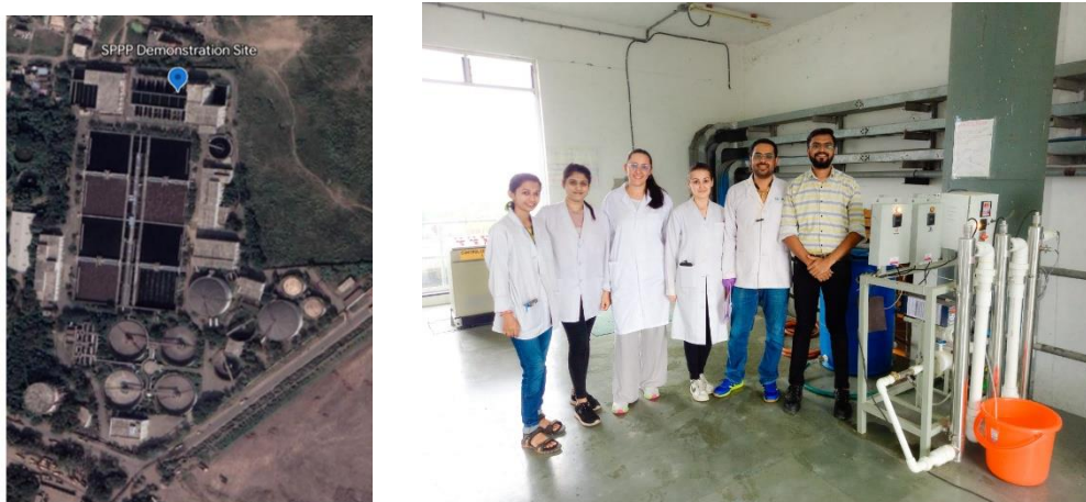
Figure 36. (Left) Bhandewadi Sewage Treatment Plant (STP) used as demonstration site for the installation of the solar powered UV-C photolytic plant (SPP) (Right) picture of the SPP plant and the researchers involved in the experiment.
