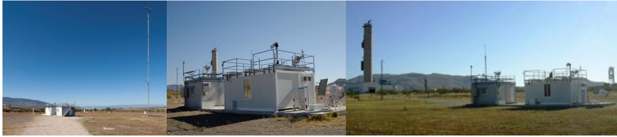
Figure 130. General view of METAS station.
